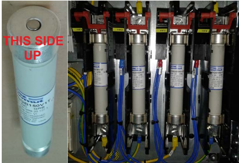
Figure 35: Correct positioning of GFDI fuses
