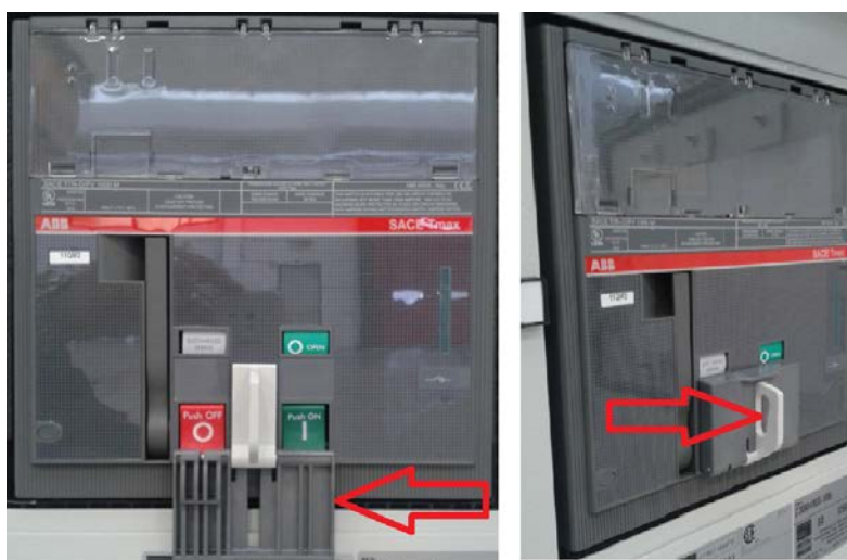
Figure 17: Pad-locking system on OFF isolator with DC or AC disconnect switch lock
