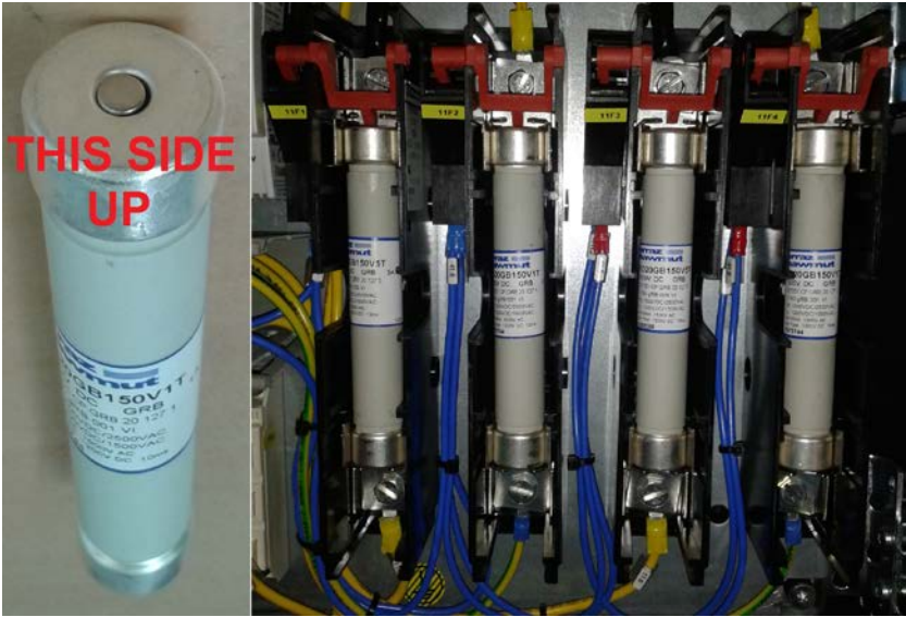
Figure 36: Correct positioning of GFDI fuse
