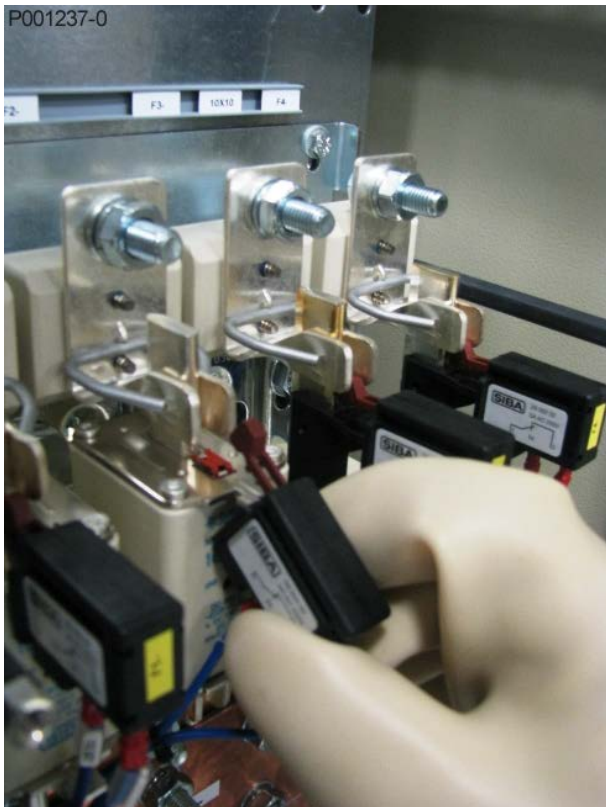
Figure 37: Extracting the fuse: microswitch disconnection and handle for removing the fuse
