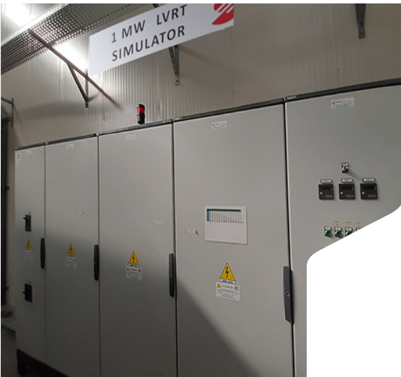
Figure 2 –LVRT facility on a 1 MW simulated network
