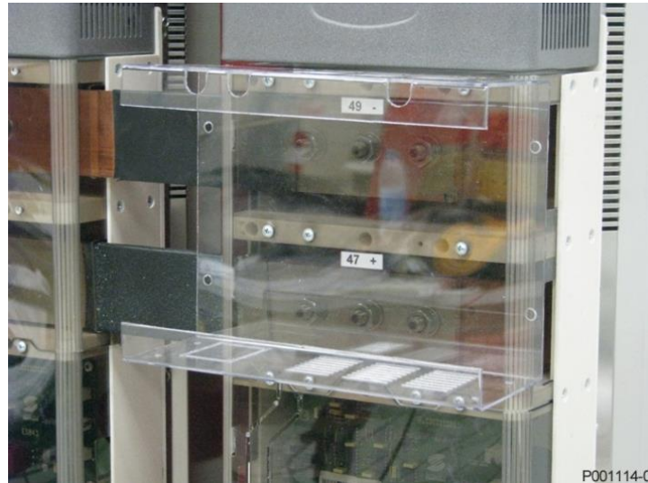
Figure 28: Cable raceway installed on the inverter module
