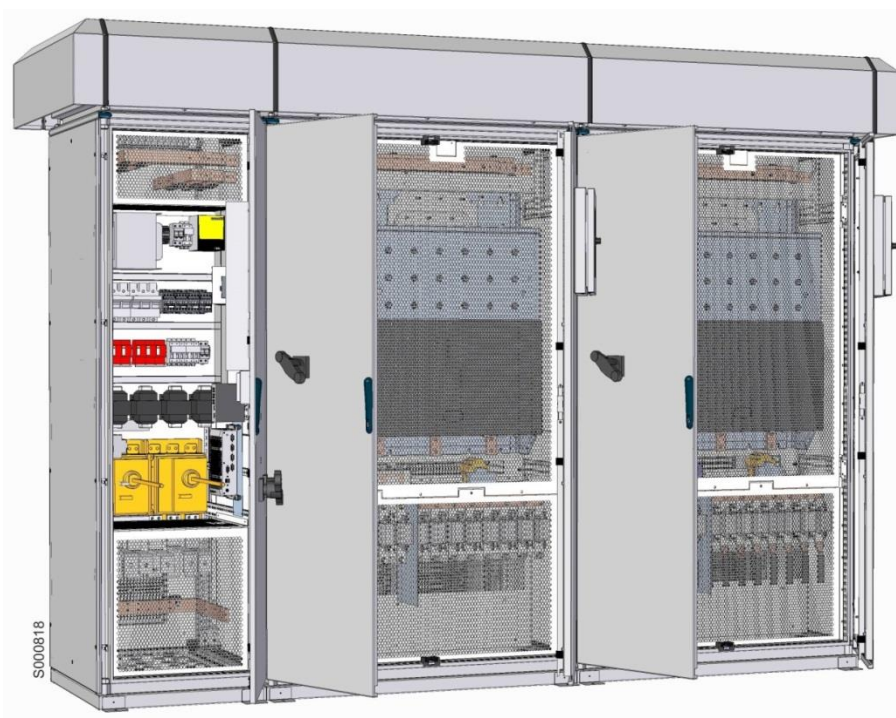
Figure 43: Protective grilles reassembled
