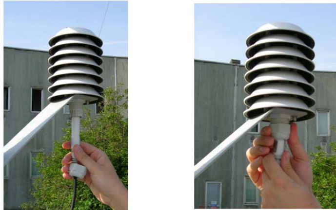
Figure 10: Installing the sensors
